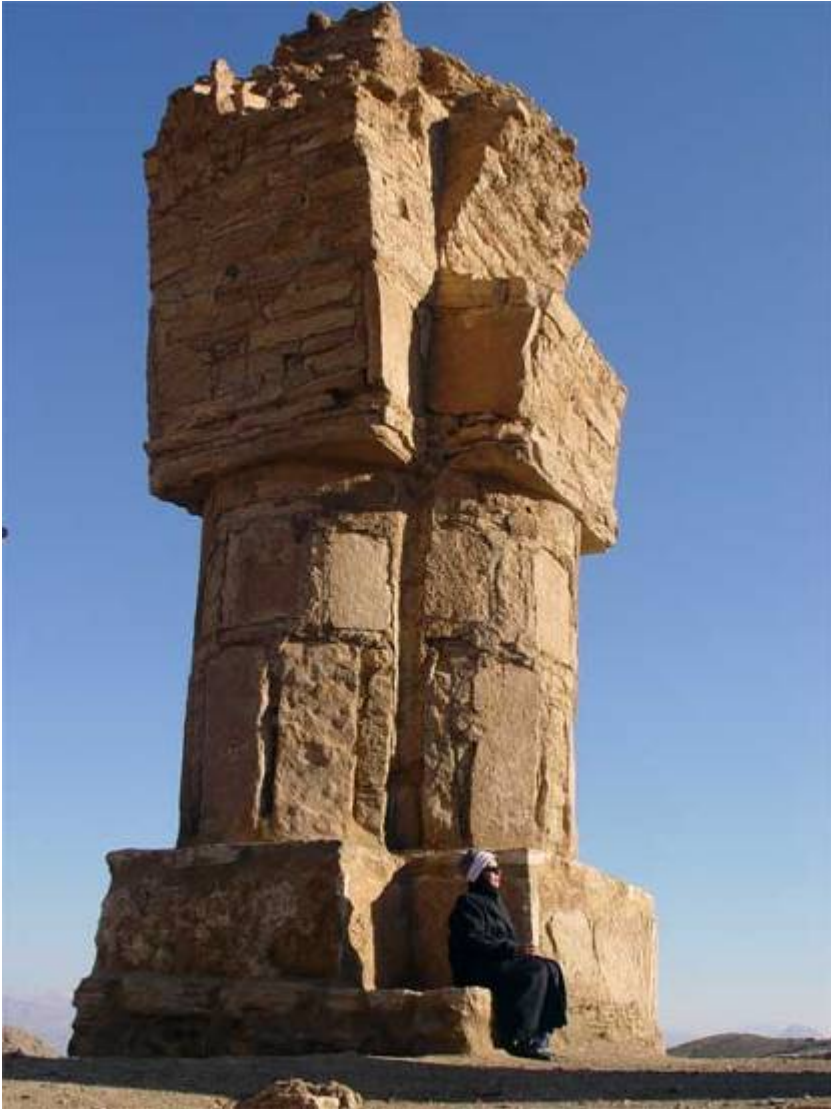
Figure 4.2: Botkhaneh Tetrapylon, the northeastern pillar
