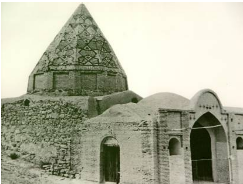
Figure 8.1: Zeinab Khatun Shrine: the southwestern side of the tetrapylon that its spans have been filled.
