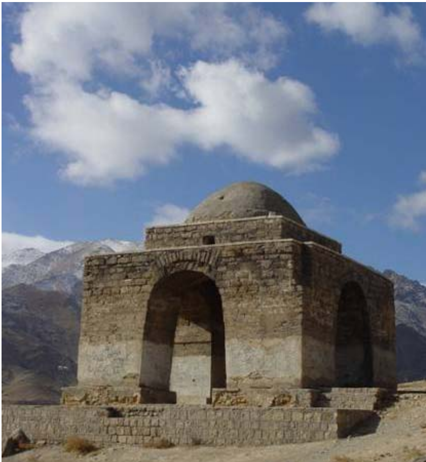
Figure 3.1: Niasar Tetrapylon, the western view
