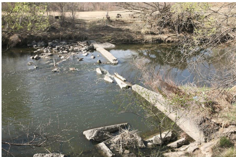
Failed concrete weir on Clear Creek
