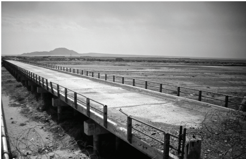
Arghestan Bridge, Kandahar province
