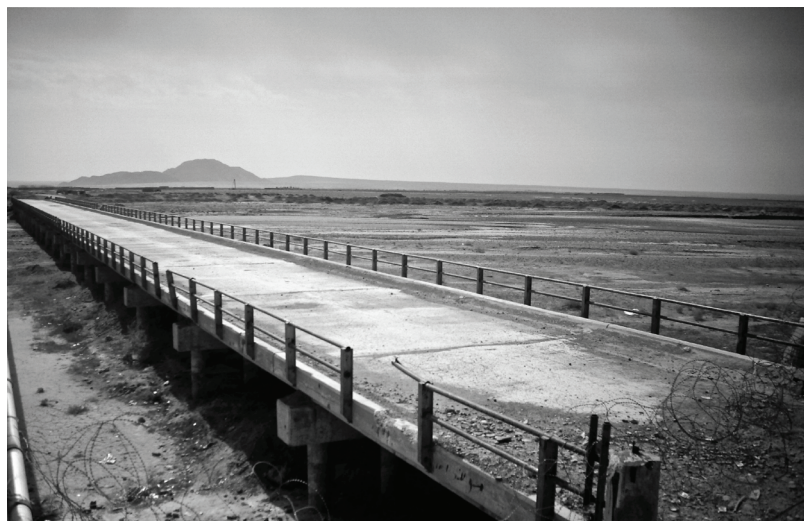
Arghestan Bridge, Kandahar province
