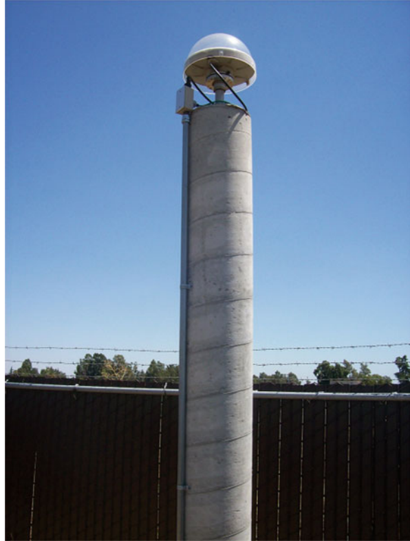
Fig. 6.1 GNSS CORS antenna on a monument pillar
