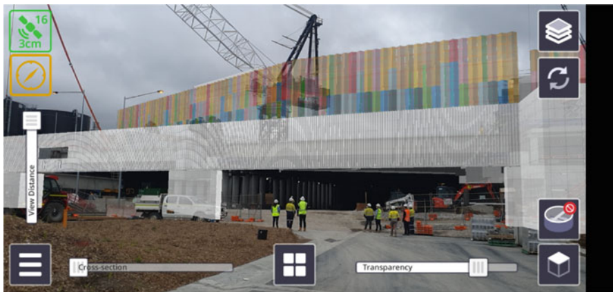
Fig. 1.7 A snapshot of SiteVision AR in real-time overlay of design data of the tunnel facade onto the existing conditions at the work location in The M4-M5 Link Tunnels project in Sydney, Australia, in 2021. Image used by permission. Courtesy of WestConnex ( westconnex.com.au )
