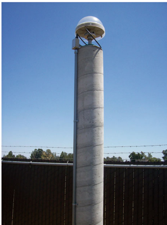
Fig. 6.1 GNSS CORS antenna on a monument pillar
