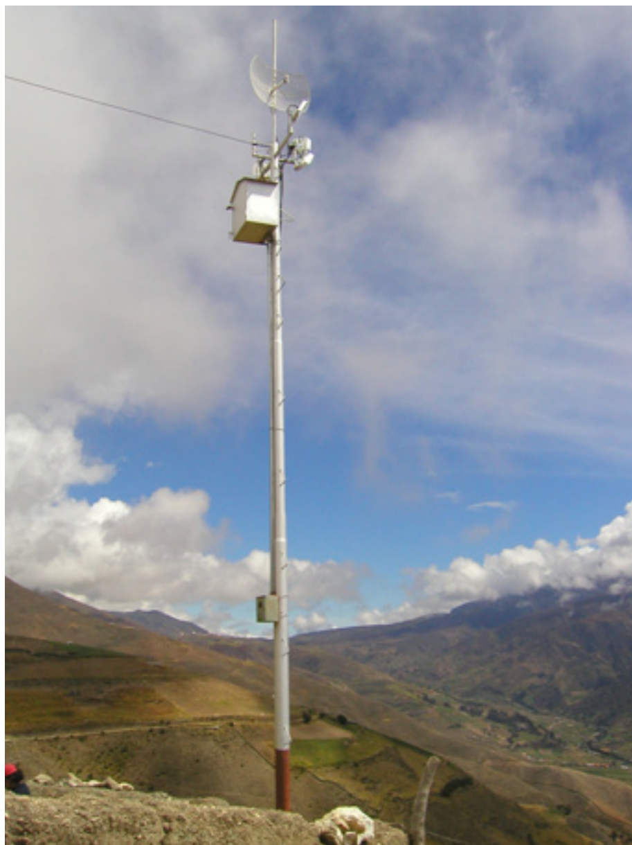
Figure 8.3: A simple self-supporting tower.
