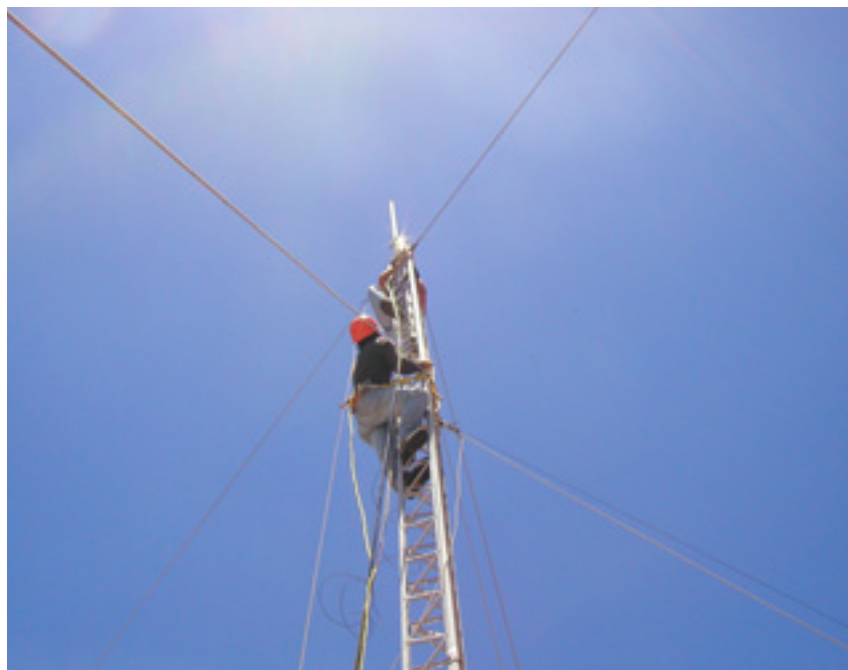
Figure 8.2: A climbable guyed tower.
