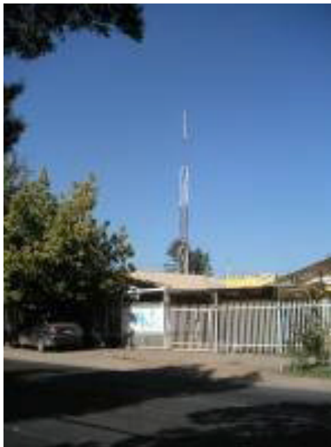
Figure 11.21: Node in southern Santiago, consisting of a 15 m tower, a Trevor Marshall 16+16 antenna, and 30 clients. The node is connected to a downtown node more than 12 km away.
