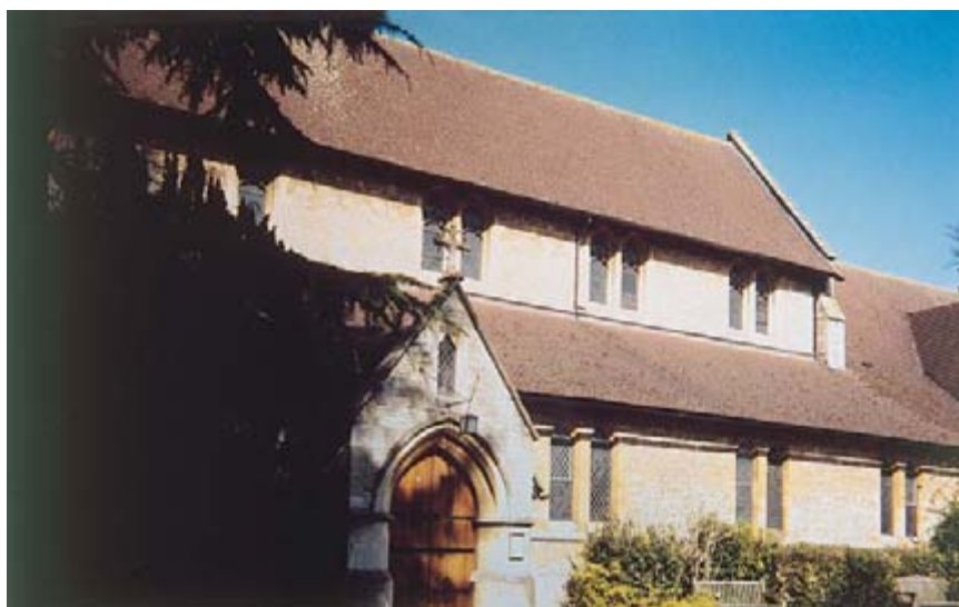
Extension to Boxmoor church
