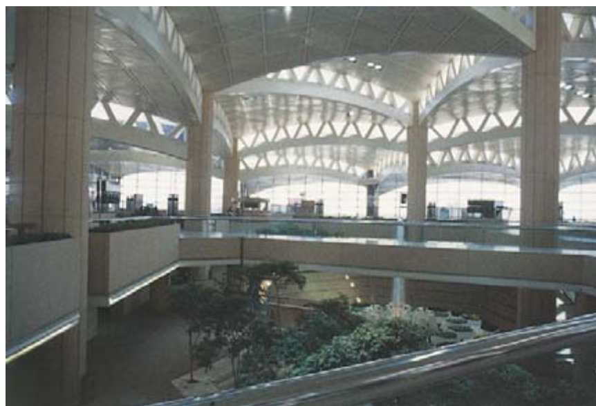
The King Khalid Airport, Riyadh, Saudi Arabia
