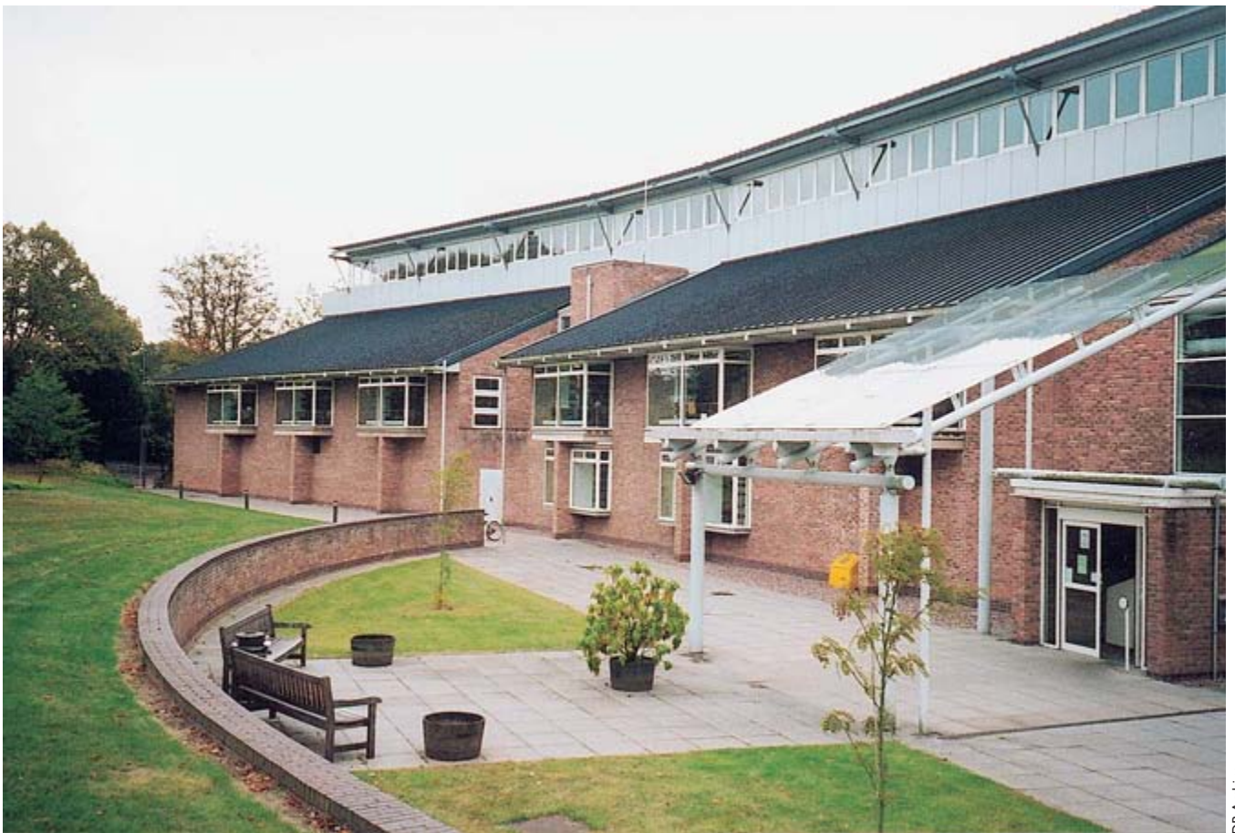
North elevation to show the projecting bays
