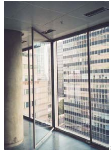
Detail of window with opening leaf
