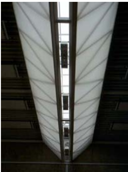
Sports hall detail of fabric diffuser
