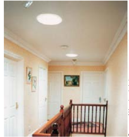
Photograph of typical light-pipe installation seen from inside the building
