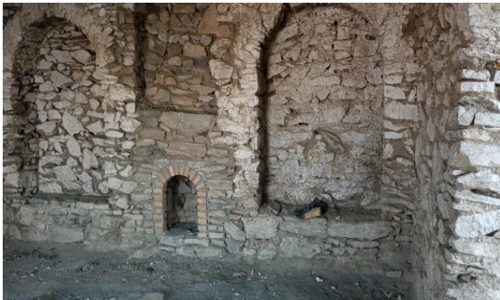
Interior pictures of the lower part of the Buddhist temple after renovation
