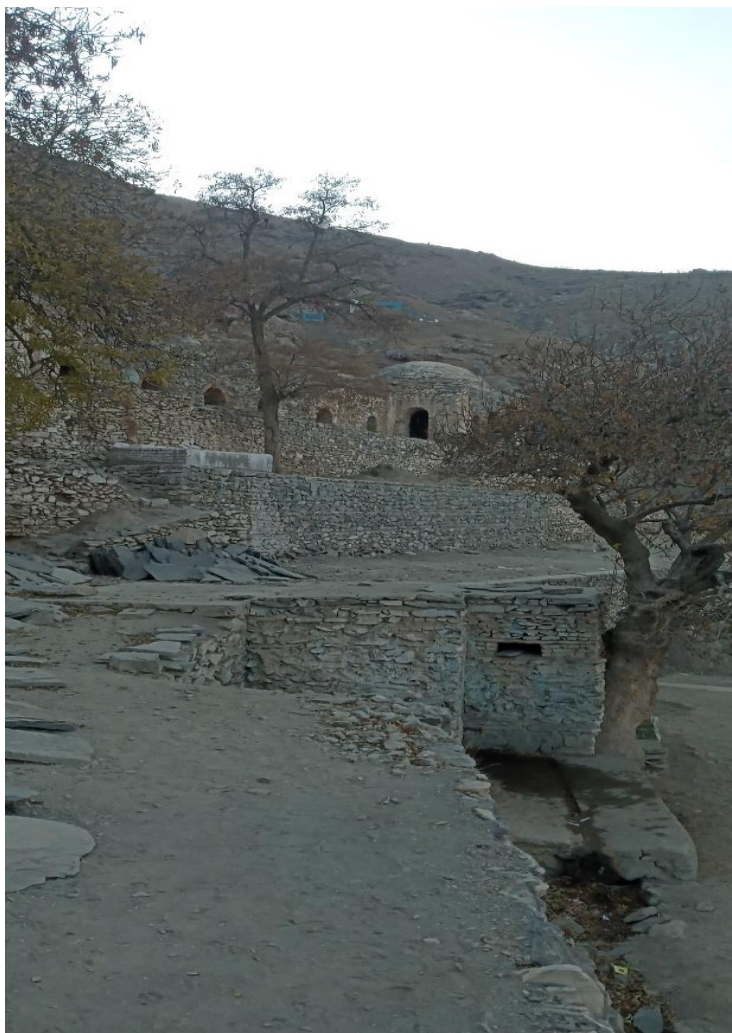
Panoramic pictures of the Buddhist temple after renovation
