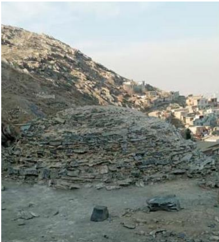
Worship hall roof panorama (covering) of the Buddhist temple during renovation
