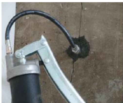
Figure 4. Injecting with a hand pump
