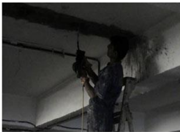
Figure 5. Epoxy injection in progress
