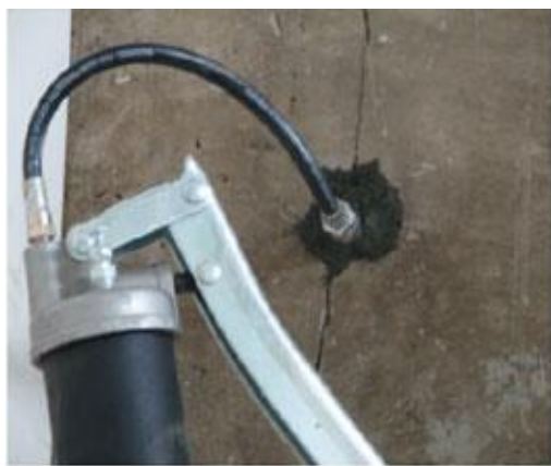
Figure 4. Injecting with a hand pump
