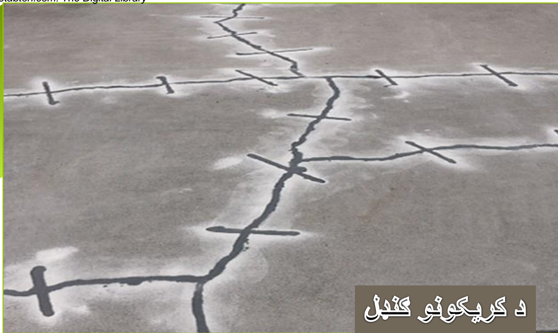
Figure 3: Stitching & Doweling
