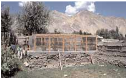
Figure 29: A type of solar dryer, made with mud walls.
