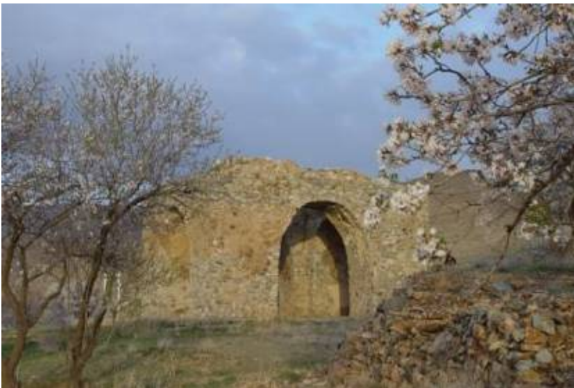
Figure 5.1: Nevis Tetrapylon, the western view
