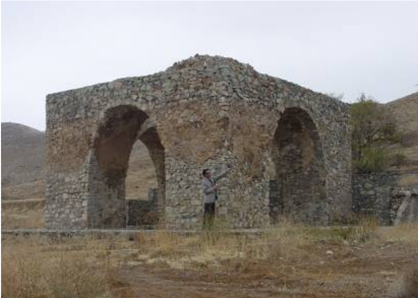
Figure 5.2: Nevis Tetrapylon, the western view
