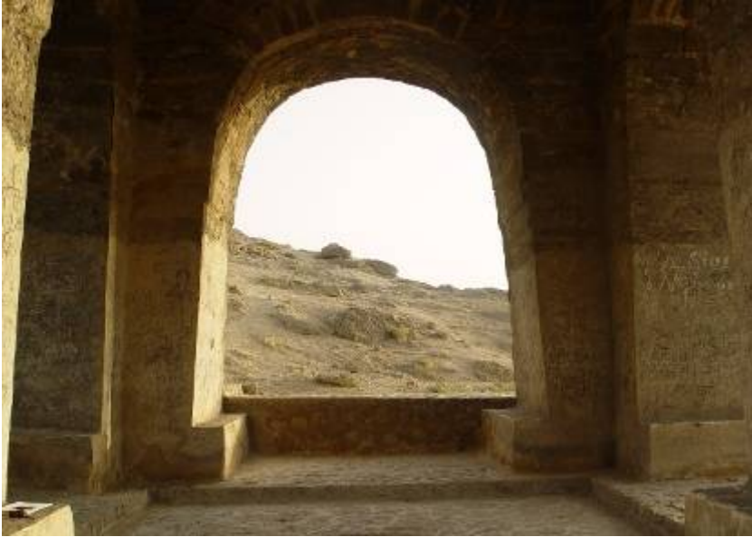
Figure 3.3: Inside Niasar Tetrapylon, the shape of pillars, and the northeastern view.
