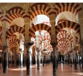
Columns in the prayer hall with two tiered arches
