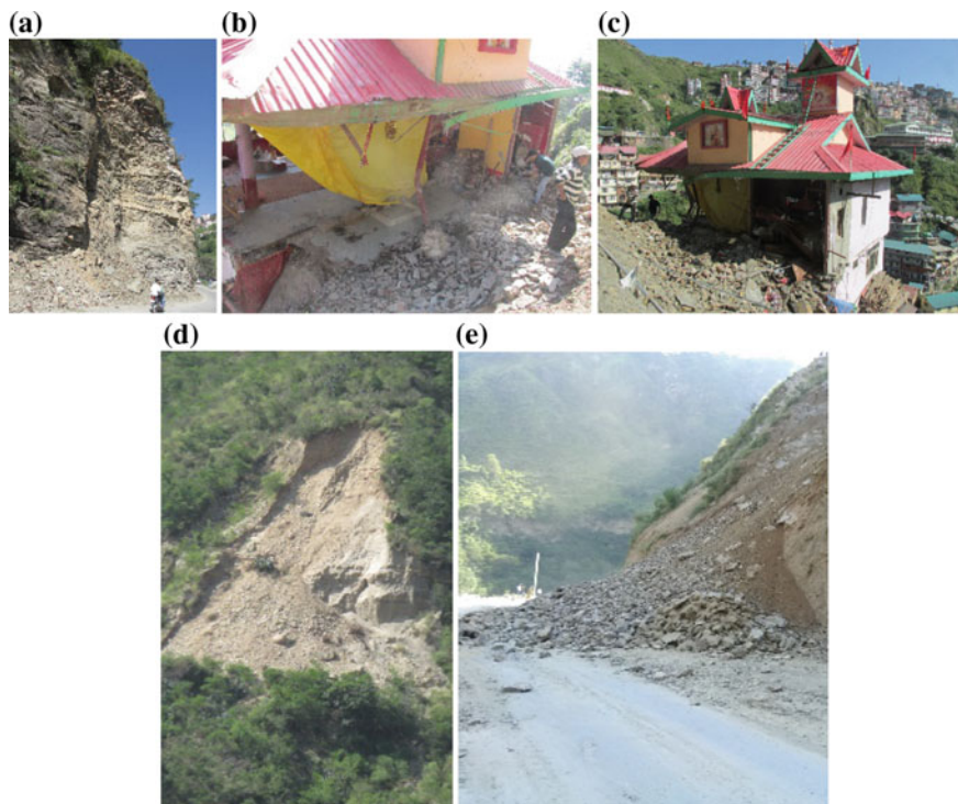
Fig. 9 a Rock slide occurred along the NH 5A in Shimla town. b and c settlements damaged due to the landslide. d and e landslide occurred along a place called Luhri located in Shimla—Rampur National Highway
