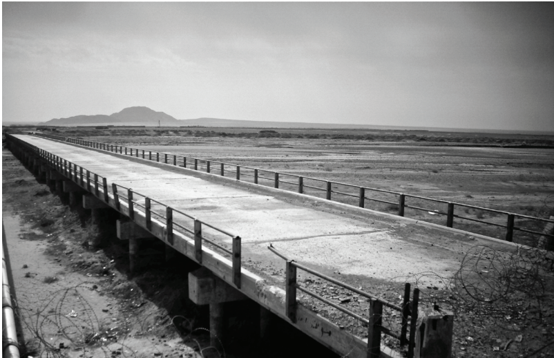
Arghestan Bridge, Kandahar province
