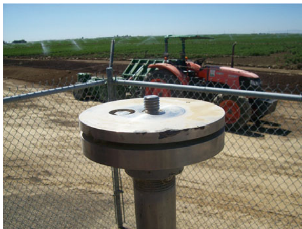
Fig. 6.4 Antenna mount without a GNSS antenna
