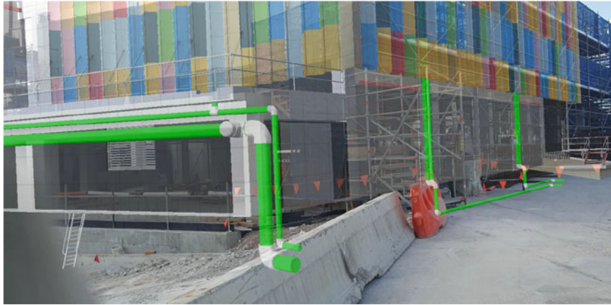
Fig. 1.6 A snapshot of SiteVision AR in real-time overlay of the design data of pipes and conduits onto the existing conditions at the work location in The M4-M5 Link Tunnels project in Sydney, Australia, in 2021. Image used by permission. Courtesy of WestConnex ( westconnex.com.au )
