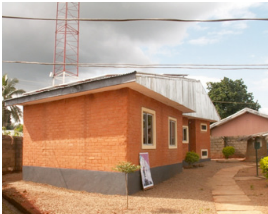
Figure 11.2: The NOC is built by locally made laterite brick stones, produced and laid by youths in Kafanchan.
