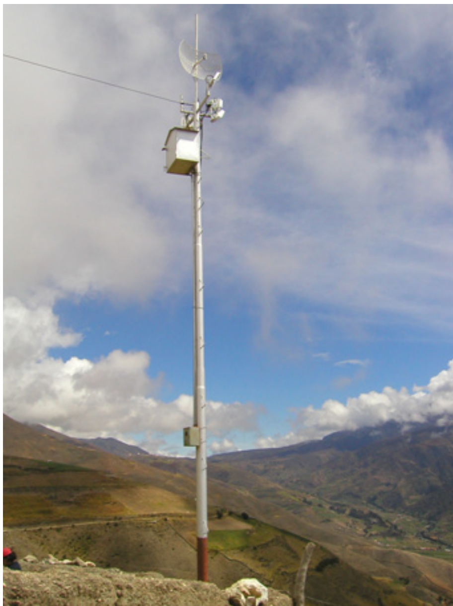
Figure 8.3: A simple self-supporting tower.
