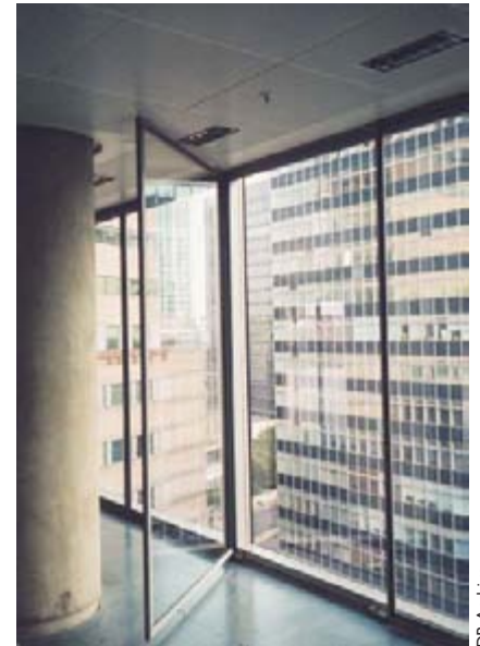
Detail of window with opening leaf
