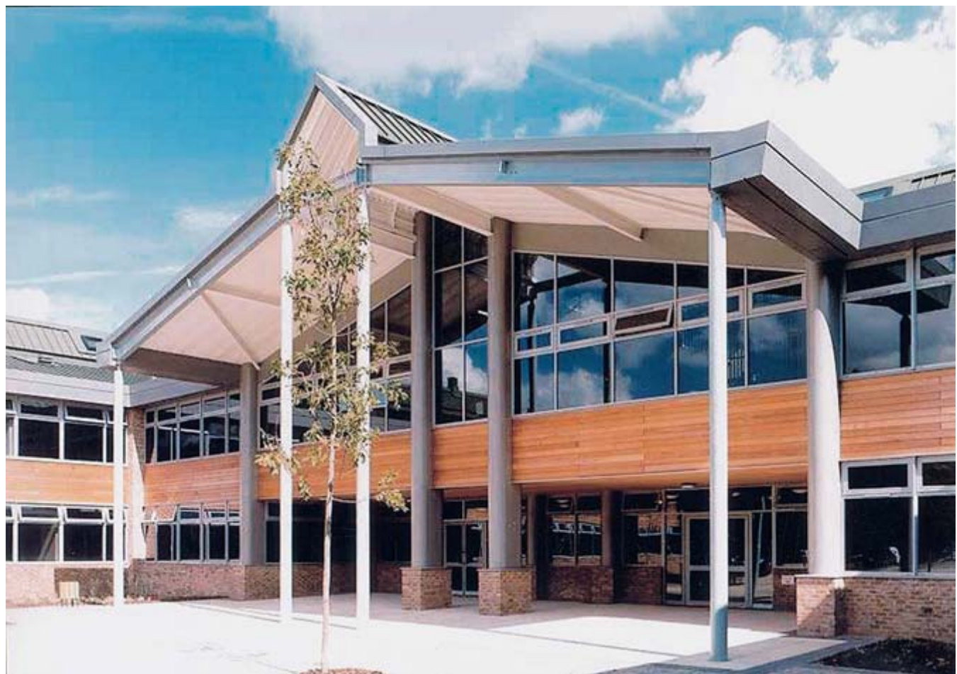
External elevation, main entrance
