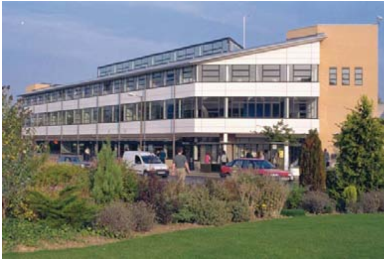
Building exterior, daylight
