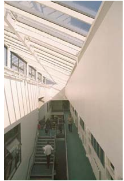
Daylighting to the atrium from roof level
