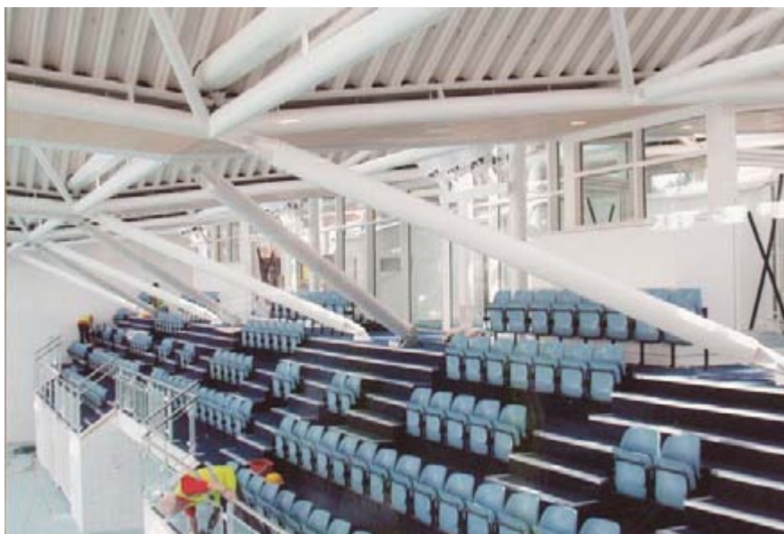
View of roof at seating level
