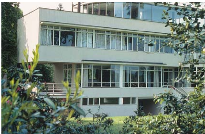
Connell Ward and Lucas House, Moor Park
