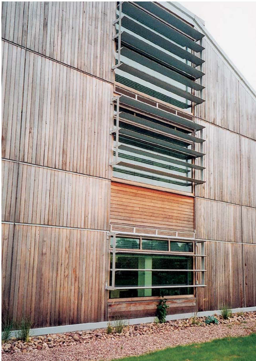
Exterior to show the application of reduced glazing and fixed louvers to southerly elevations
