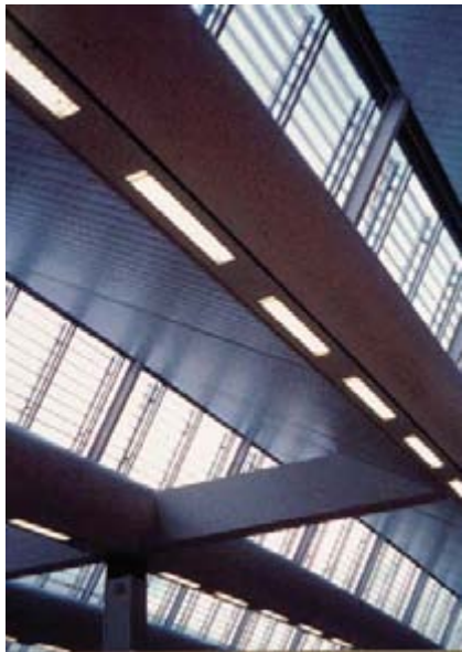
Detail of roof lighting
