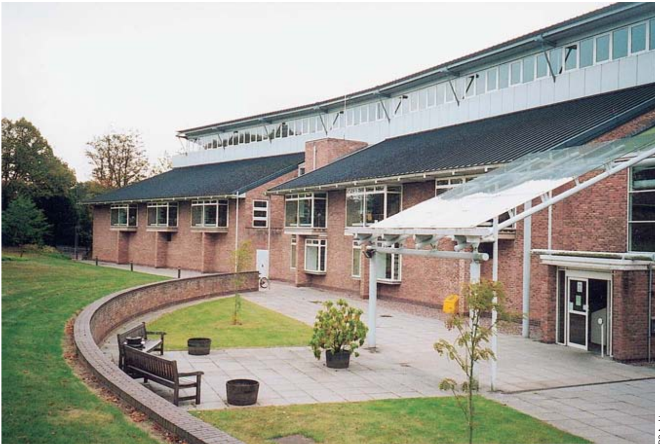
North elevation to show the projecting bays
