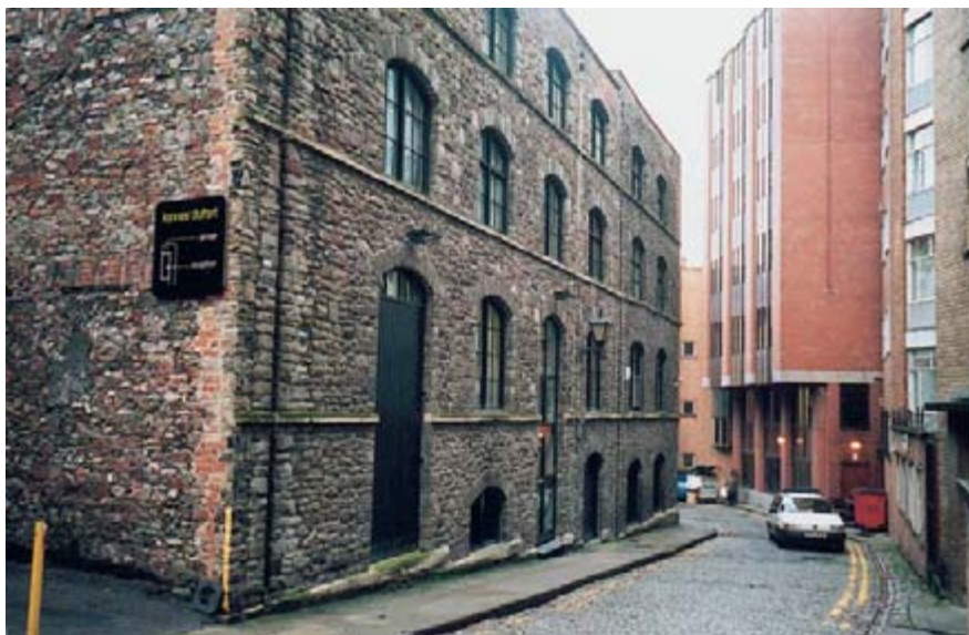
The exterior of the building
