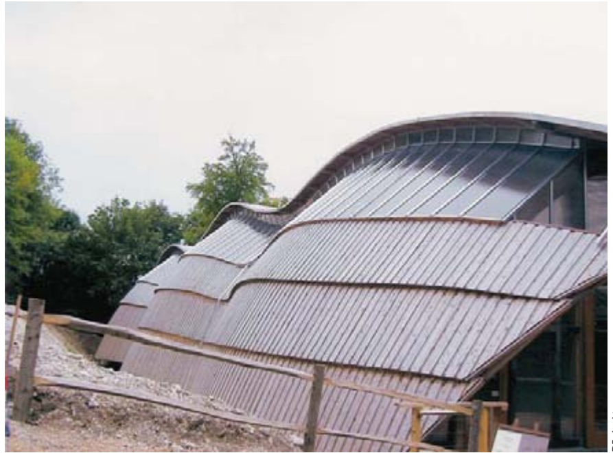
View of the exterior timber walling and high level daylight sheeting
