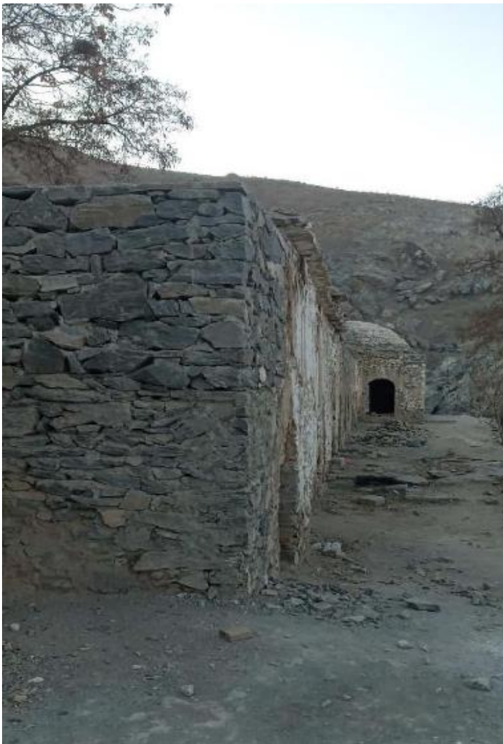
Front elevation Pictures of the Buddhist temple after renovation from the east
