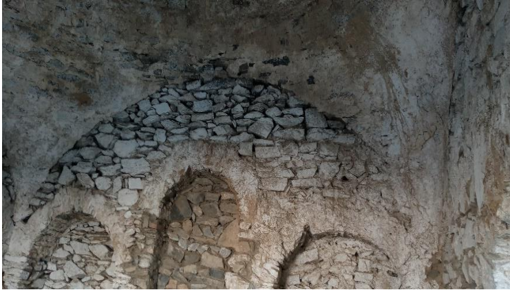
Interior pictures of the upper part of the Buddhist temple after renovation
