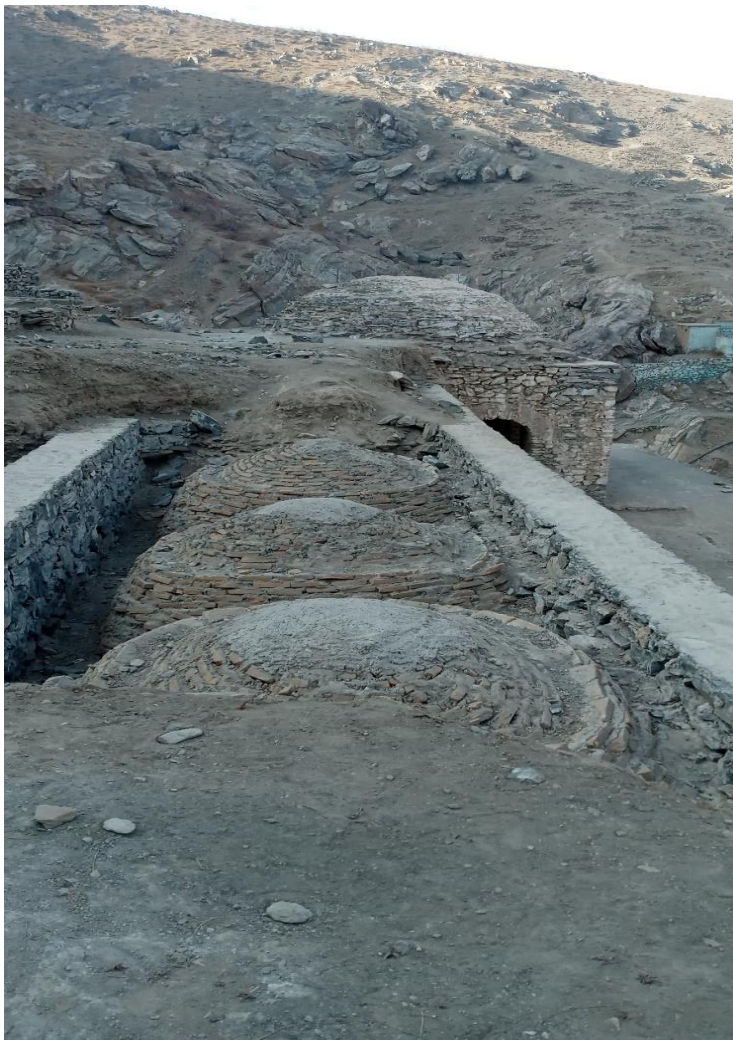
Roof panorama (covering) of the Buddhist temple during renovation
