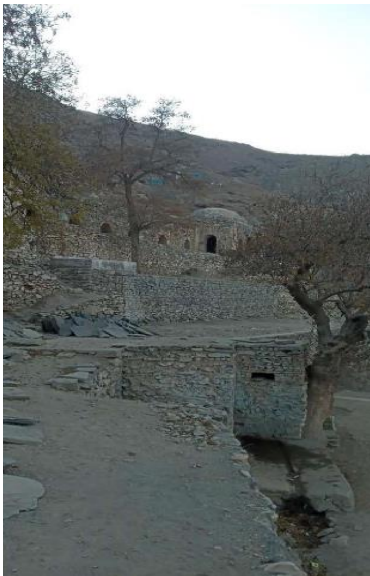
Front elevation Pictures of the Buddhist temple after renovation from the east
