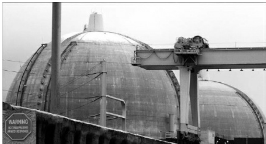
FIGURE 13–10 The nuclear power plant at San Onofre, California.
