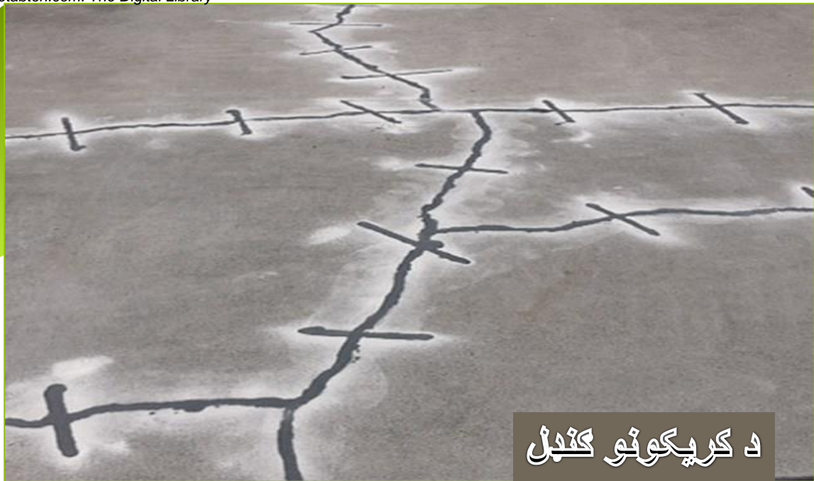
Figure 3: Stitching & Doweling
