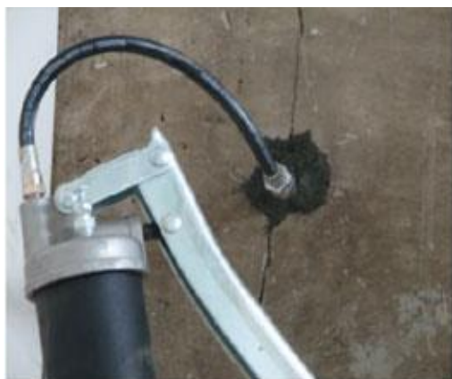
Figure 4. Injecting with a hand pump
