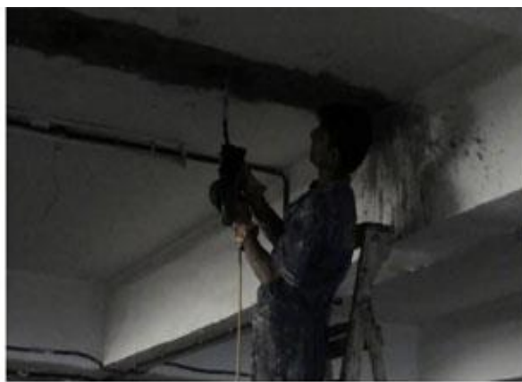
Figure 5. Epoxy injection in progress
